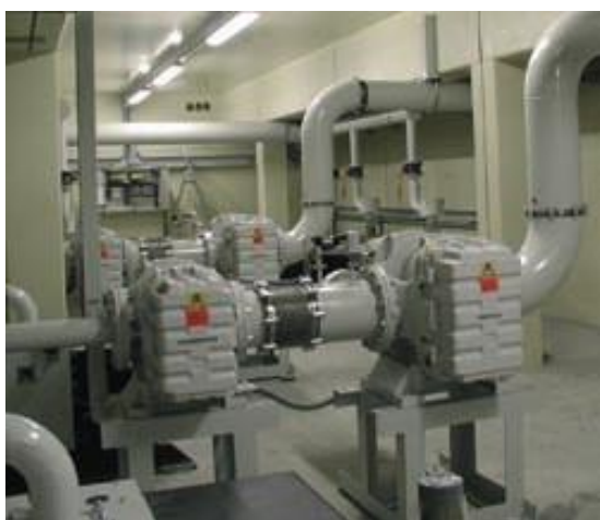
3-stage pumping set for 2 x 12.000 m 3 /h ▼ in inscription technology
